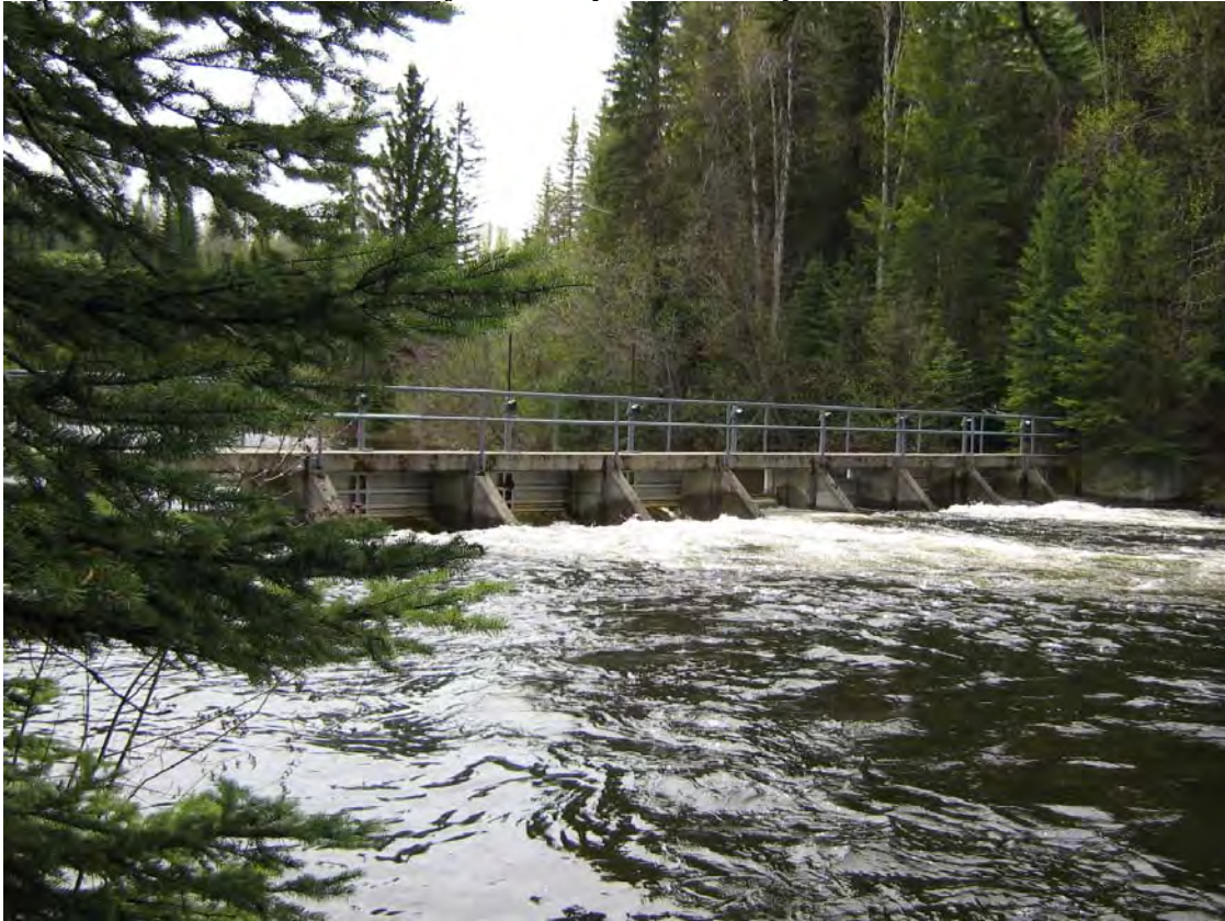
Figure 10: Downstream view of McKinley Dam in May 2008.
